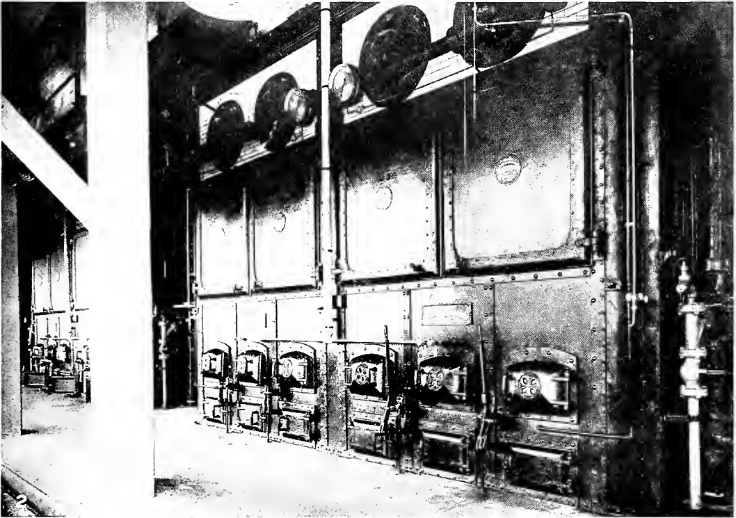
1. Shipping D'Olier boiler plant equipment to the canal. 2. The boilers installed at Miraflores power plant. (D'Olier Engineering Company, Philadelphia, Pa.)
